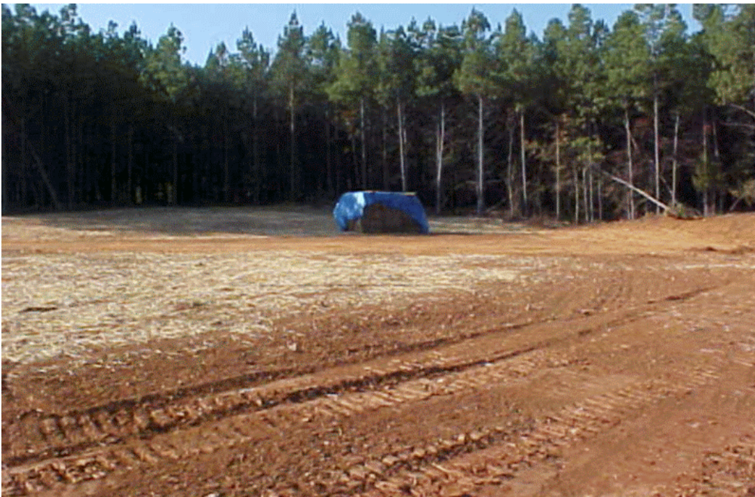
Photograph #22: From top of hill above E08N looking north-northwest. The blue tarp is covering hay bails used to help control erosion.
