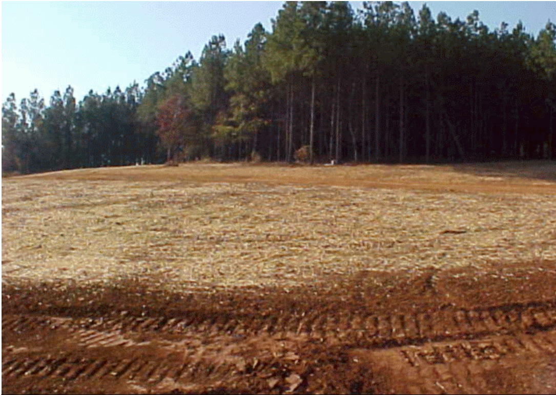
Photograph #23: From above E08N, looking west. The top of the hill has been leveled and hay spread to control erosion.
